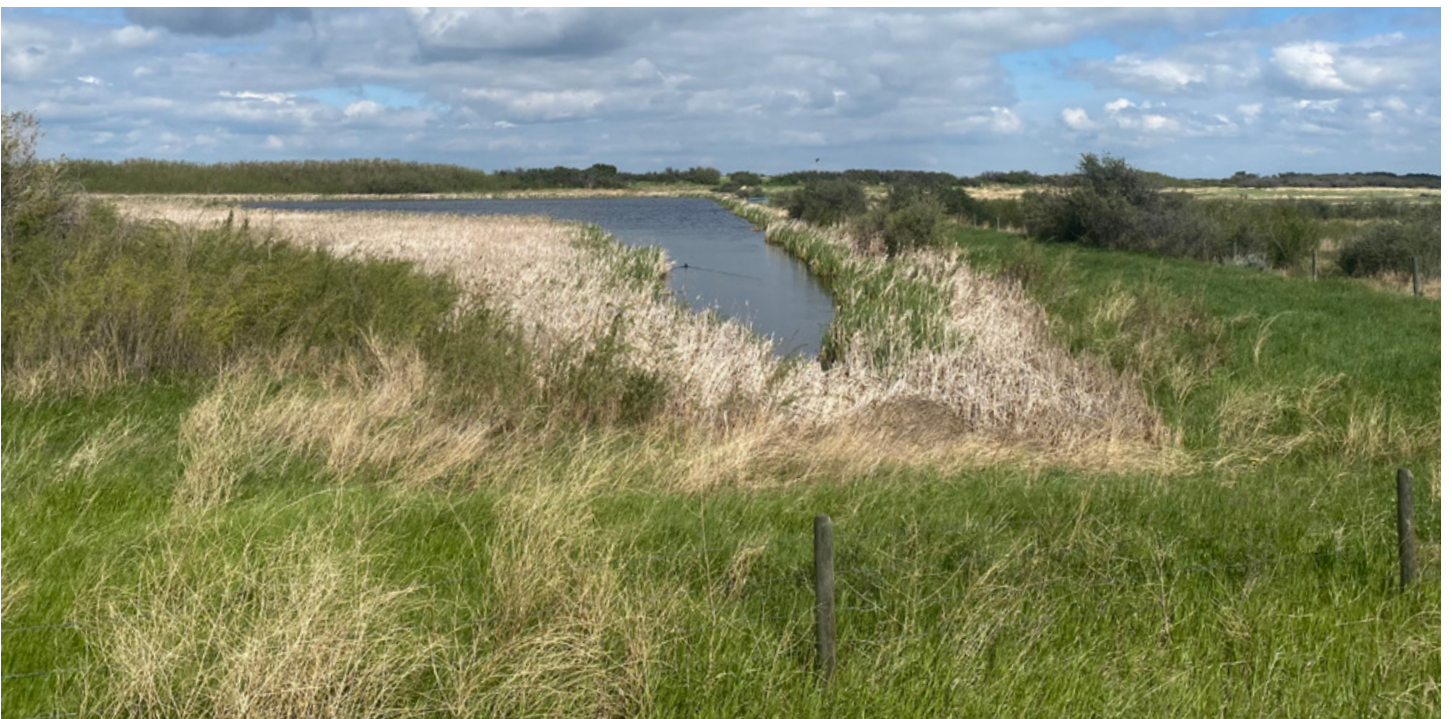
Finnegan Field is the last wetland complex before the water runs into the Red Deer River near Finnegan ferry. The structures in this complex are more than 30 years old and in need of repair. PF Calgary will hire local contractors to make sure these wetlands remain on the landscape.
